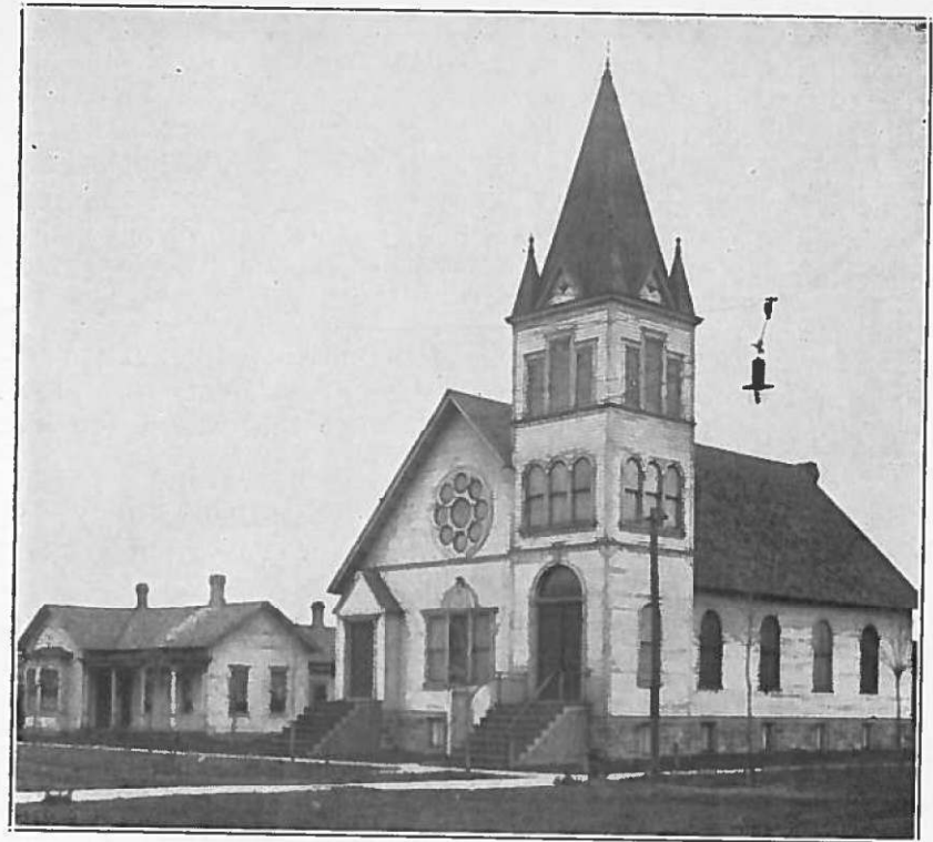
The Church with its rebuilt tower
